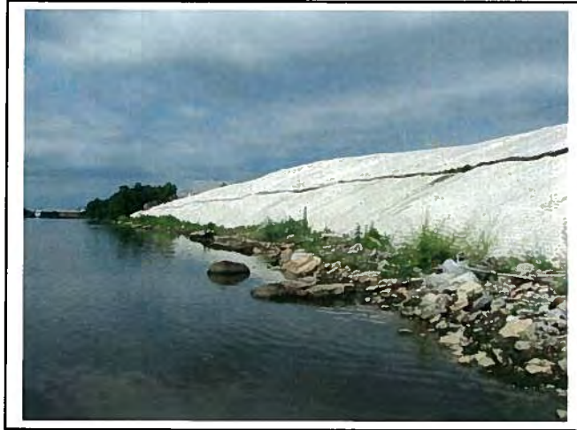
Upstream end facing downstream.
