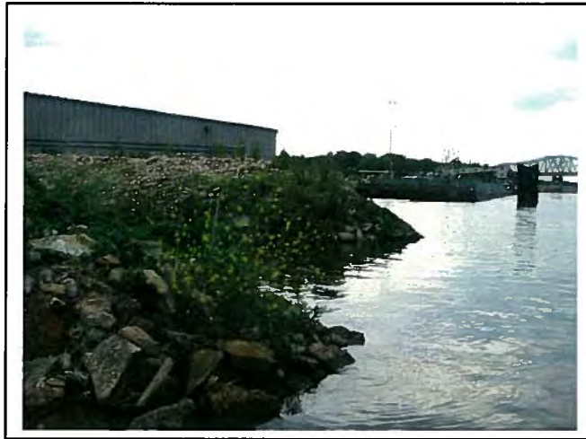
Upstream end facing downstream.
