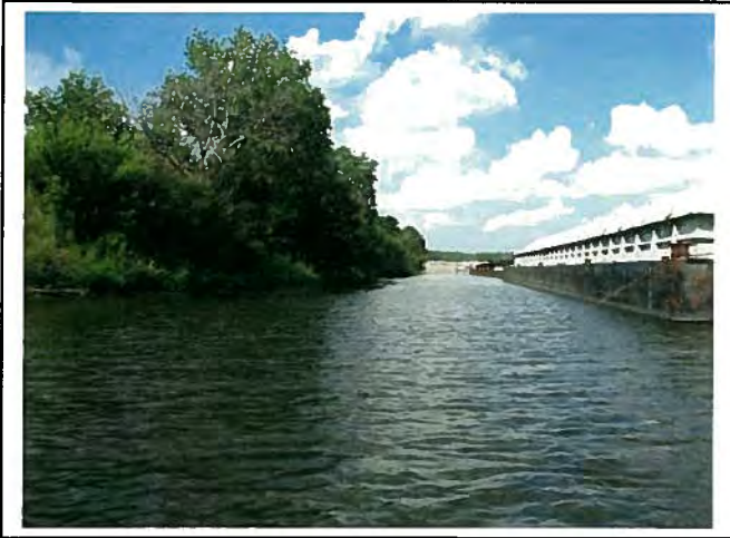
Middle of zone facing upstream.
