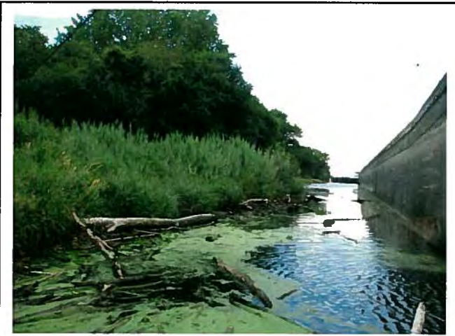
Downstream end facing upstream.
