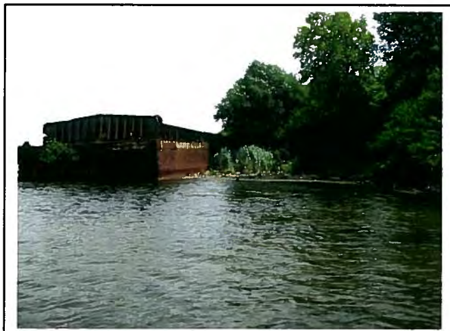
Downstream end facing upstream.
