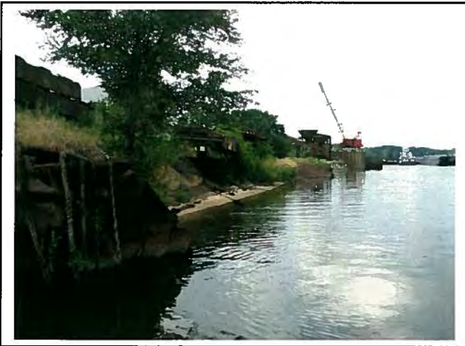
Downstream end facing upstream.
