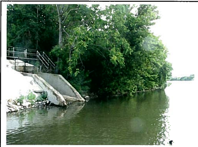
Downstream end facing upstream.
