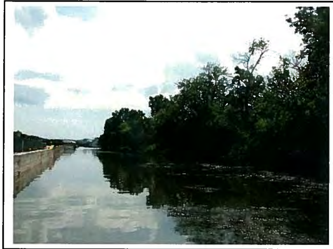
Upstream end facing downstream.
