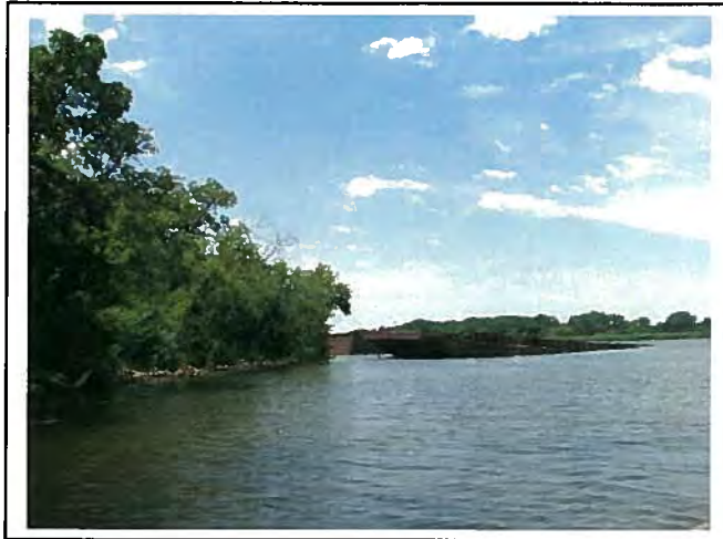
Upstream end facing downstream.
