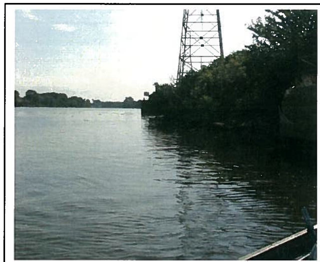
Downstream end facing upstream.
