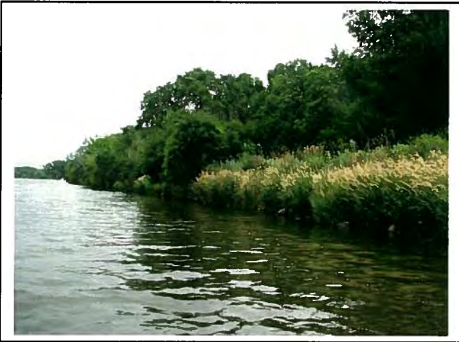
Downstream end facing upstream.
