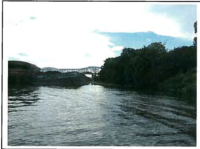
Upstream end facing downstream.
