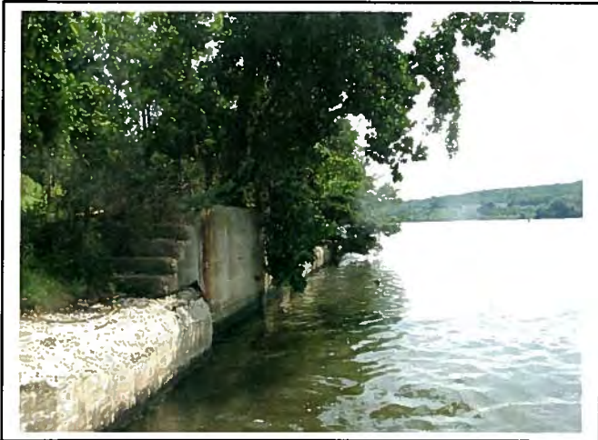
Middle of zone facing upstream.
