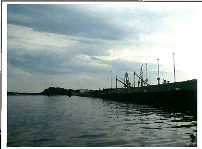
Middle of zone facing upstream.
