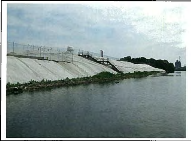
Middle of zone facing upstream.
