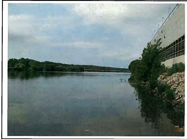
Upstream end facing downstream.
