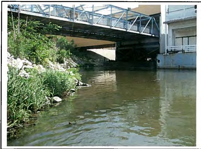
Middle of zone facing upstream.
