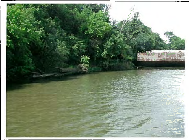
Middle of zone facing upstream.
