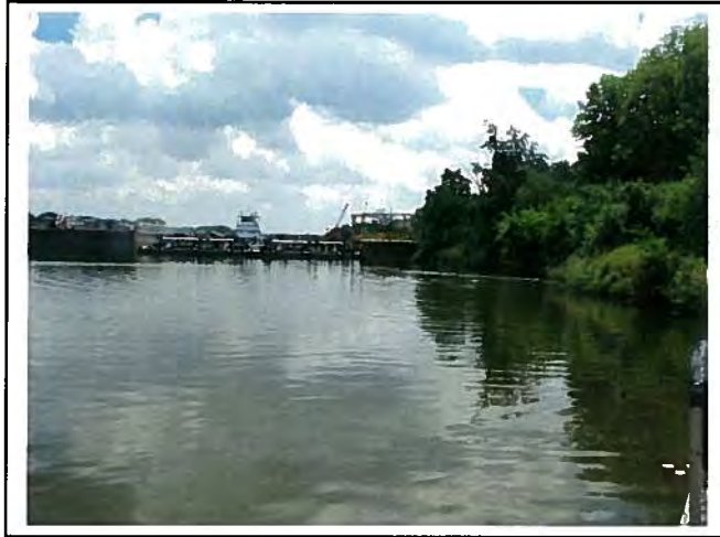
Upstream end facing downstream.
