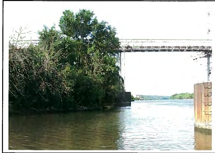
Upstream end facing downstream.
