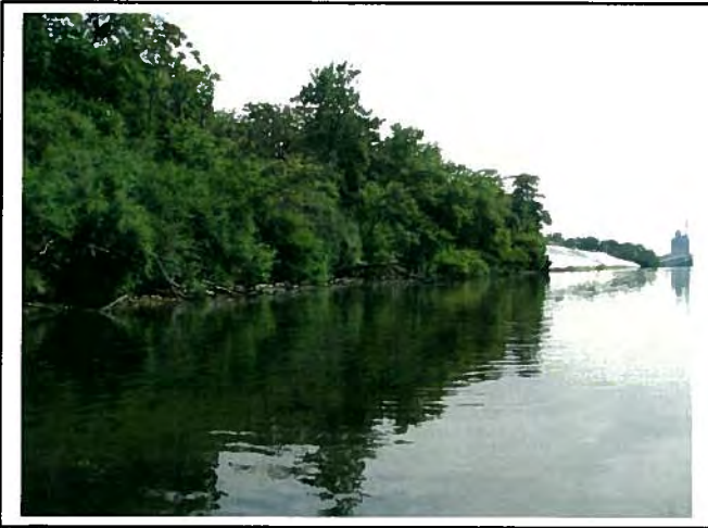
Downstream end facing upstream.
