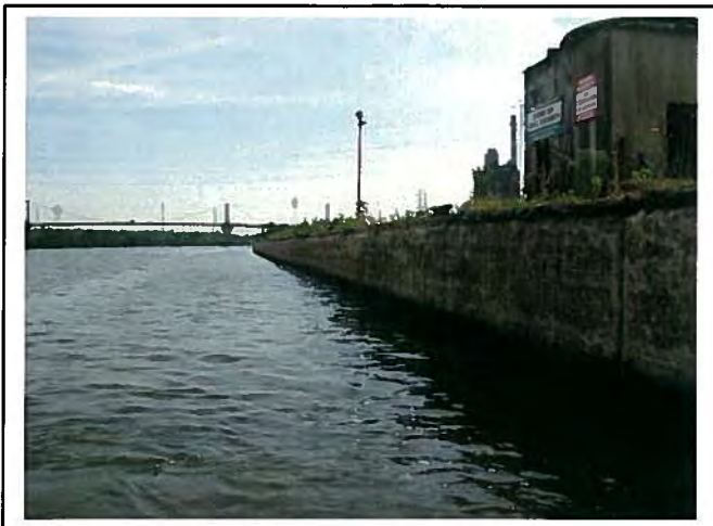
Middle of zone facing upstream.
