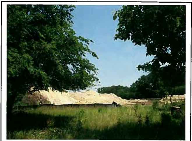
Construction activities adjacent to this location.
