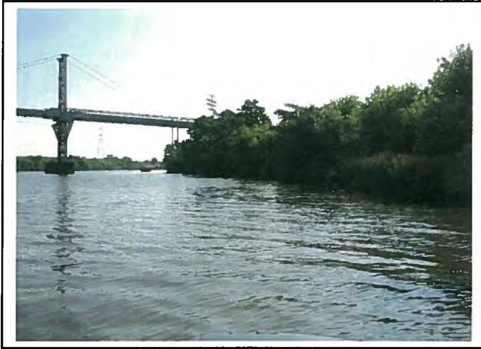
Middle of zone facing upstream.
