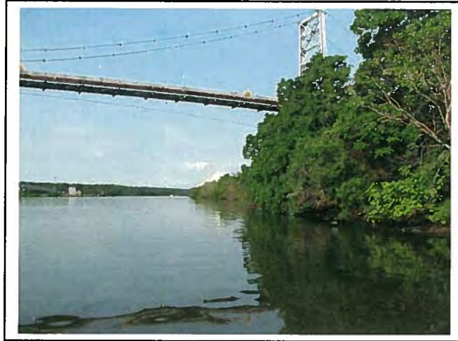
Upstream end facing downstream.
