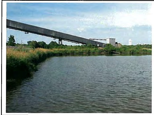
Upstream end facing downstream.
