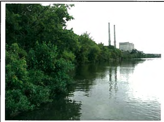
Downstream end facing upstream.
