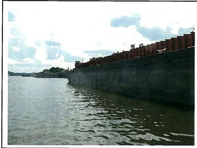
Upstream end facing downstream.
